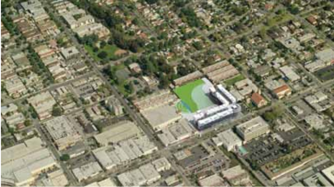
Aerial Looking North
