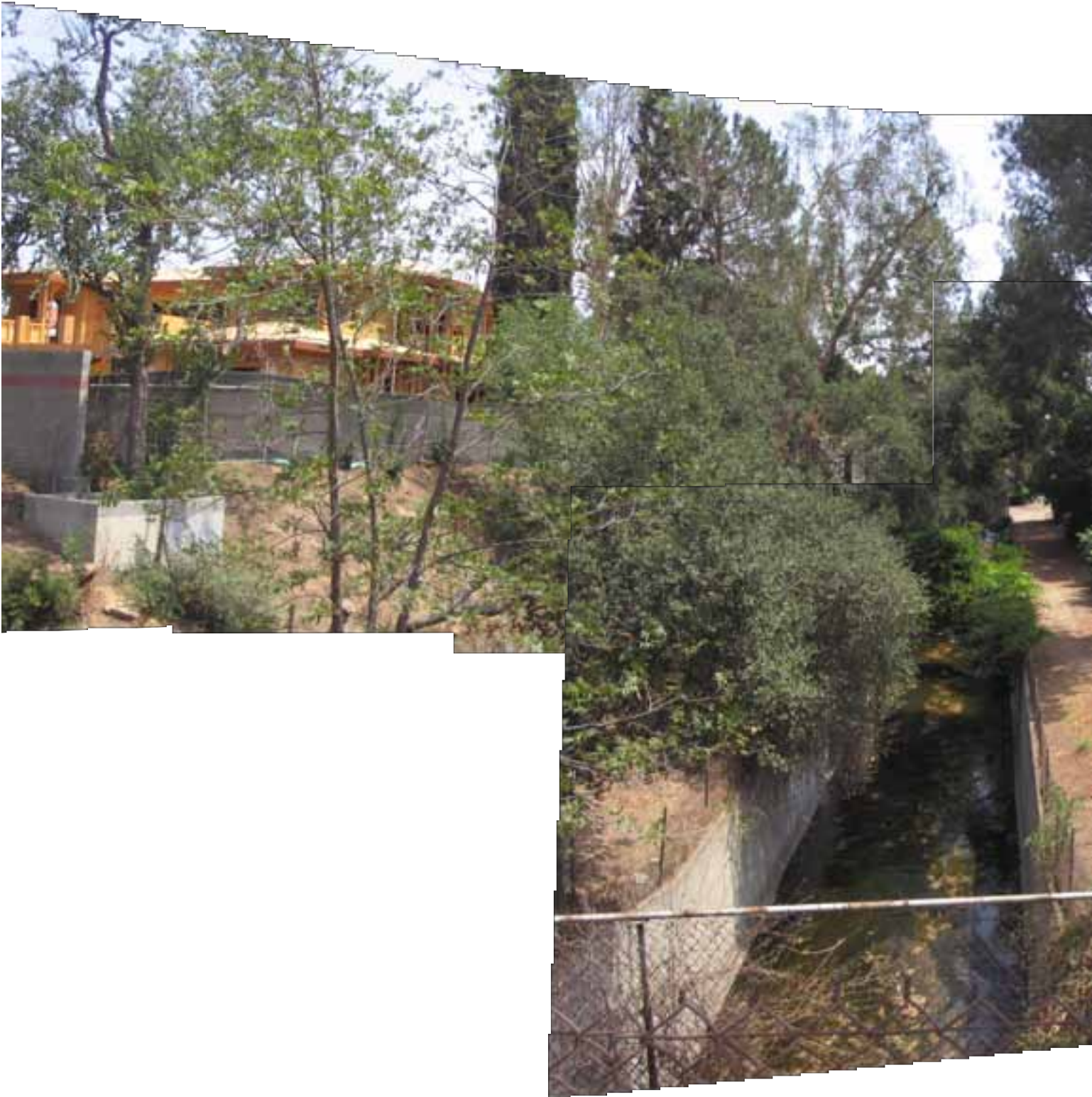
the culvert, looking south towards the site
